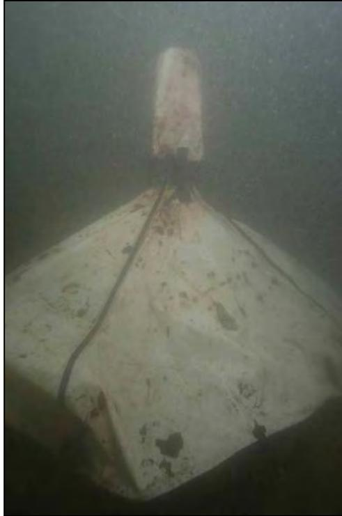
Figure 9.21. Oil catchment tent deployed on *Arizona* (NPS Photo by Brett Seymour).
