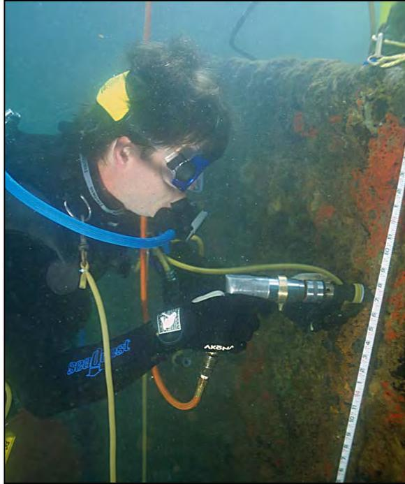
Figure 5.17. Drilling through USS *Arizona*'s exterior concretion in preparation to measuring  $E_{\text{corr}}$  and pH (NPS Photo by Brett Seymour).
