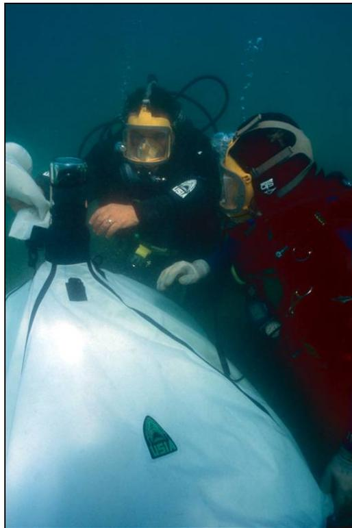
Figure 9.22. Oil catchment tent deployment on *Arizona* (NPS Photo by Brett Seymour).
