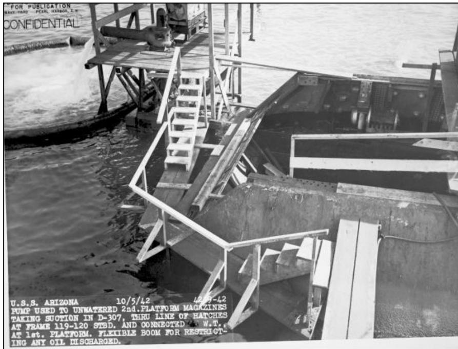
**Figure 3.12. Pump and platform used to unwater second platform magazines, Space D-307, Frame 119-120, October 5, 1942 (USS Arizona Memorial Photo Archive).**
